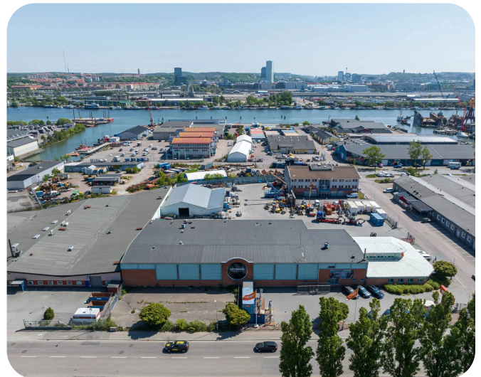
Light industrial - Gothenburg
